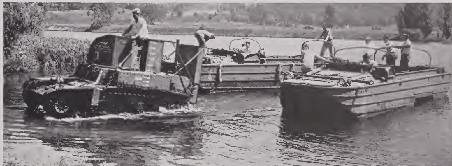
FIGURE 62. Wet ferry completed: light tank climbing to dry land.
